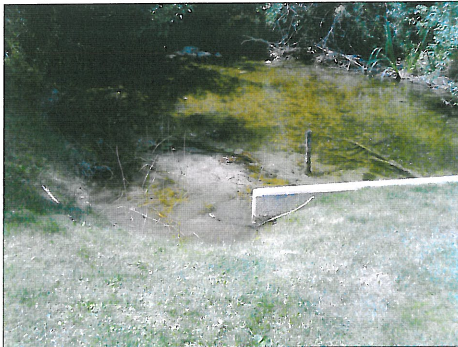
AT DAM LOOKING WEST TOWARDS OUTLET
