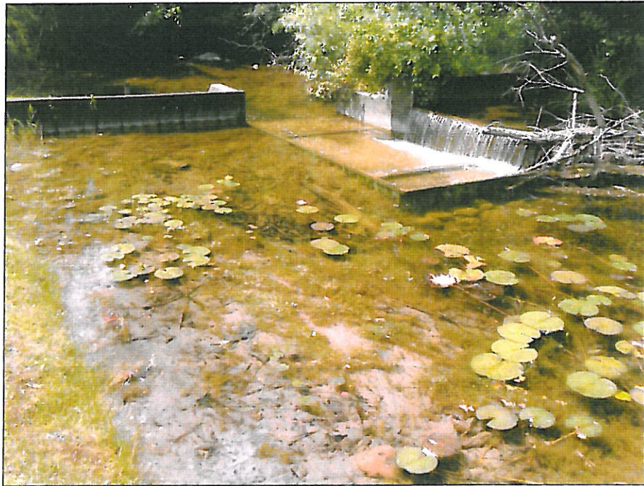
LOOKING WEST TOWARD DAM
